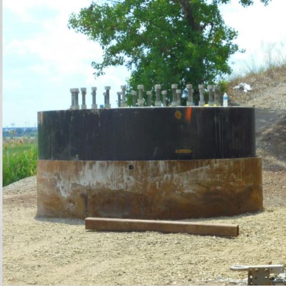
Transmission Pole 2B Foundation Installation Completed
