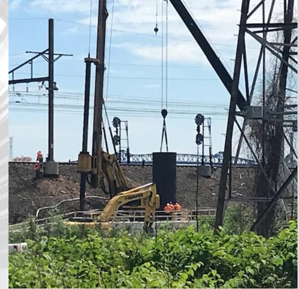
Transmission Pole 2A Setting a 8-Foot Deep Casing for Foundation
