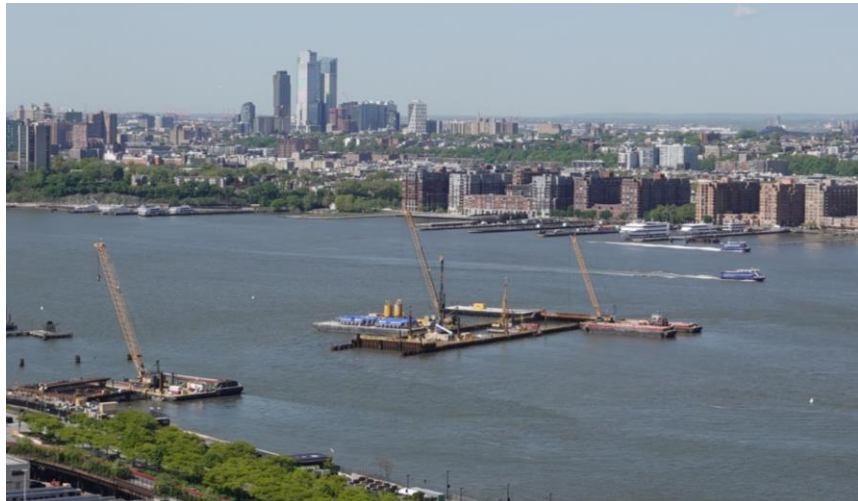
The HRGS cofferdam and construction barges in the Hudson River.
