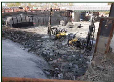
October 28, 2025 Drilling of blast holes (Looking West)
