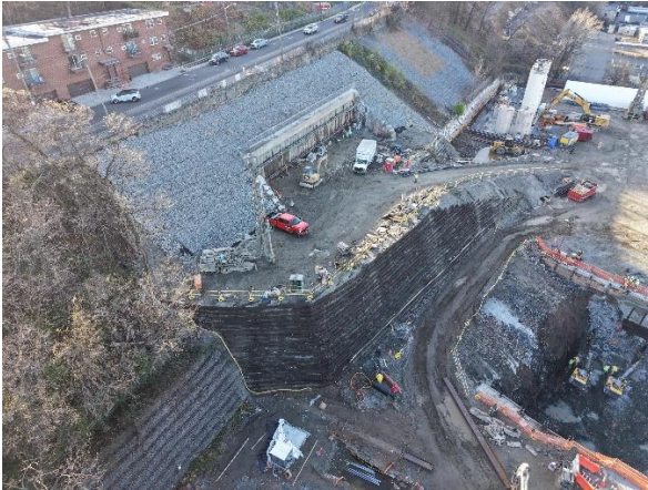
Construction of the tunnel boring machine portal launch box in North Bergen, NJ.
