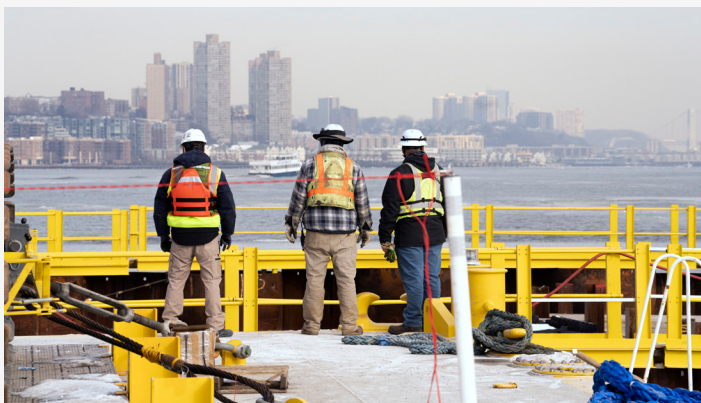
Hudson River Ground Stabilization
