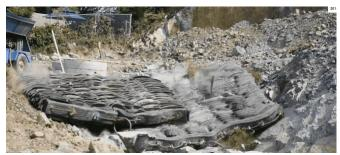
Blasting mats play a vital role in protecting both workers and the surrounding community by containing blasting activity, preventing debris from leaving the blast zone, and helping to reduce noise and dust.
