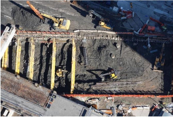
Excavation is underway on the 80-foot-deep hole where the new section of the concrete casing is being built.
