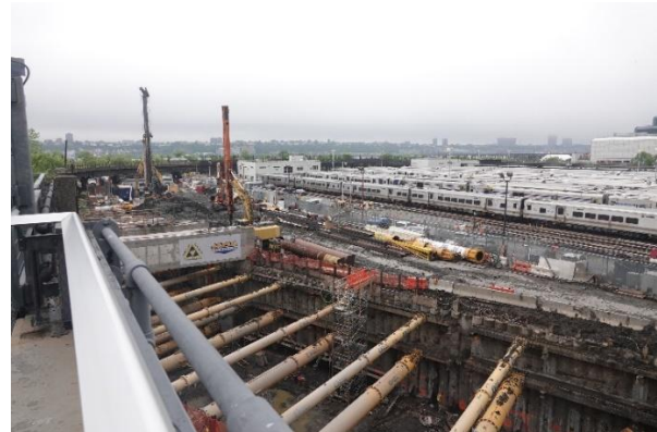
Once excavation and dewatering is complete, the team will build the new section of the concrete casing, then re-fill the hole.
