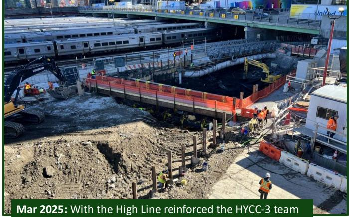
is now focused on excavating an 80-foot-deep hole to build the tunnel box.
