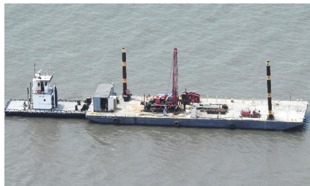
HRGS construction barge working in the Hudson River
