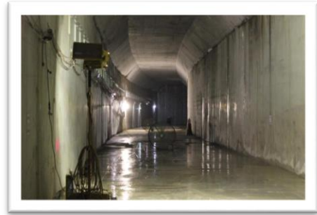
Figure 3: Completed Section of the Hudson Yards Concrete Casing
