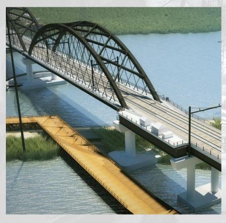
» Fixed, two-track bridge » 50 feet clearance above mean high-water »2.33 mile project area »25 multi-level cars to provide a greater than 10% increase in peak hour passenger capacity »New signals and power supply » **Demolition** of existing bridge »90 mph speed limit
