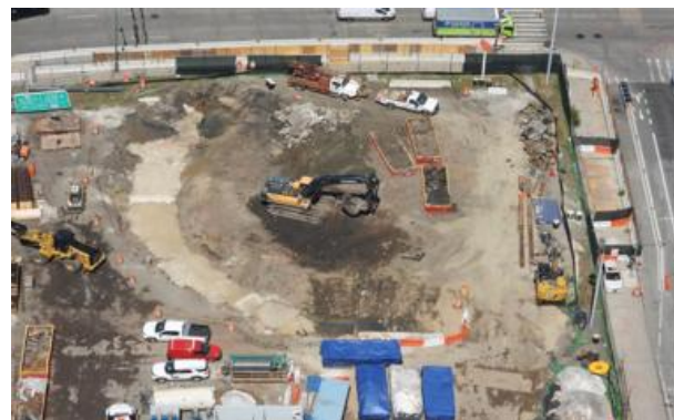
Figure 9: July – 12 th Ave Shaft pre trenching operations
