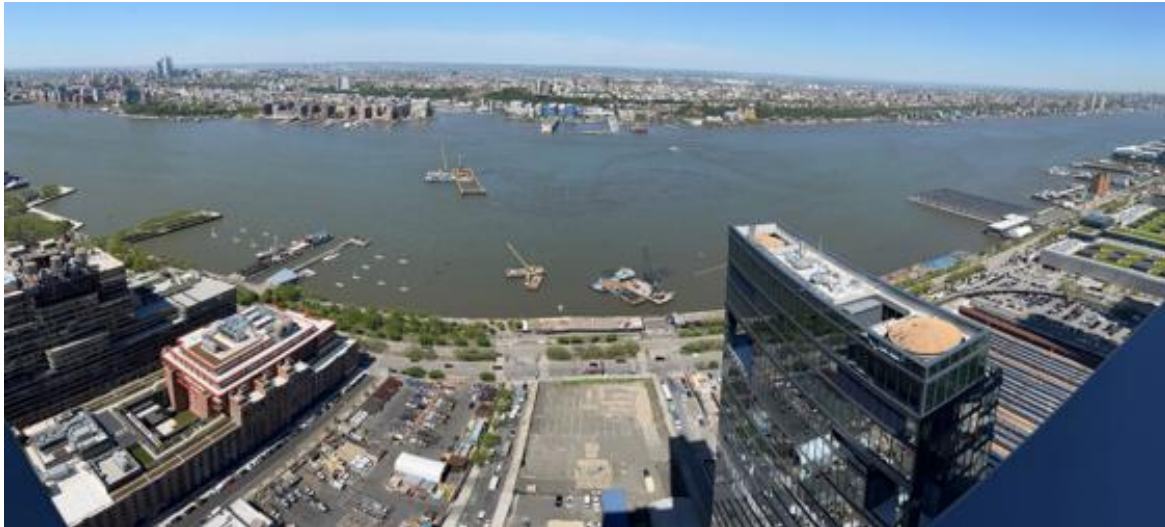
Figure 5: April – Aerial View of Work Area Location (Looking West)
