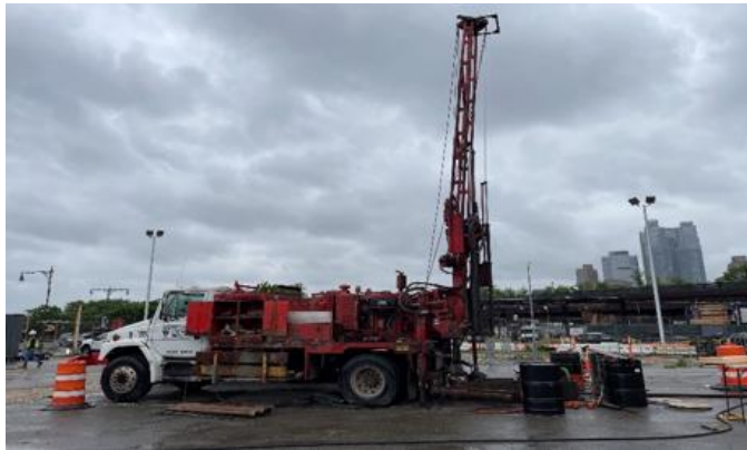
Figure 7: May – Geotechnical boring (Looking North)
