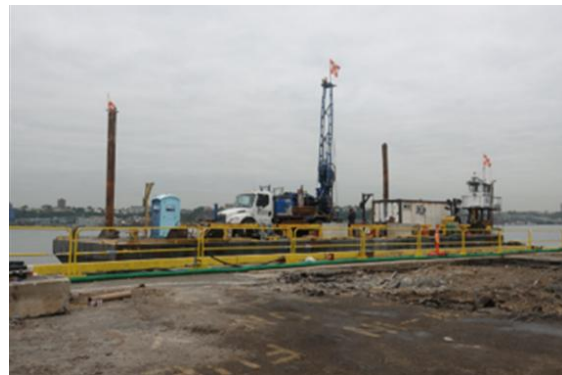
Figure 11: September – Over-Water Borings
