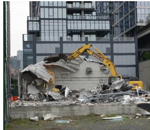
Figure 6: May – Demolition of Quonset Hut
