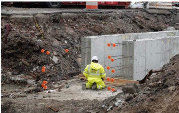
Figure 10: August – 12 th Ave Shaft Guide Wall Installation
