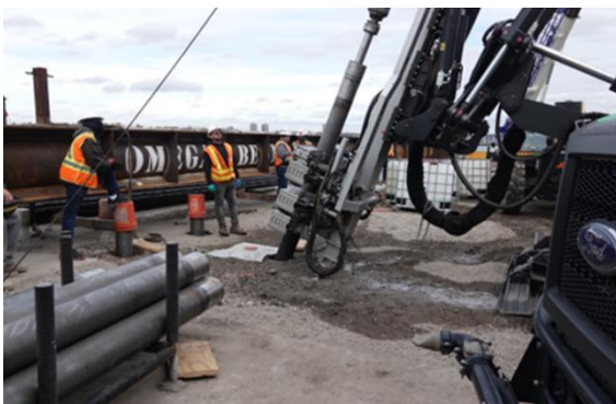
Figure 12: October – Installation of freeze pipe/grout sleeves
