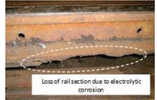
Corroded Rails
