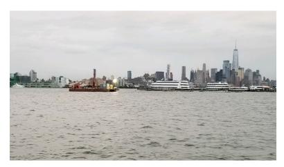
A barge mounted drill rig recently commenced drilling to investigate the Hudson River bottom, and land-based drill rigs will work along the NJ Surface Alignment in Secaucus and North Bergen, the Palisades Portal Area adjacent to Tonnelle Avenue, the Palisades Tunnel alignment, and in other areas near the New Jersey waterfront. In Manhattan, drill
