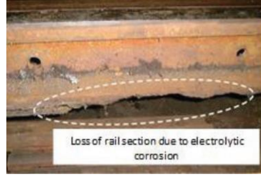
Corroded Rails
